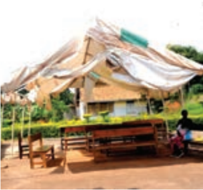
The waiting shed at Mpigi Health Center IV, before...
